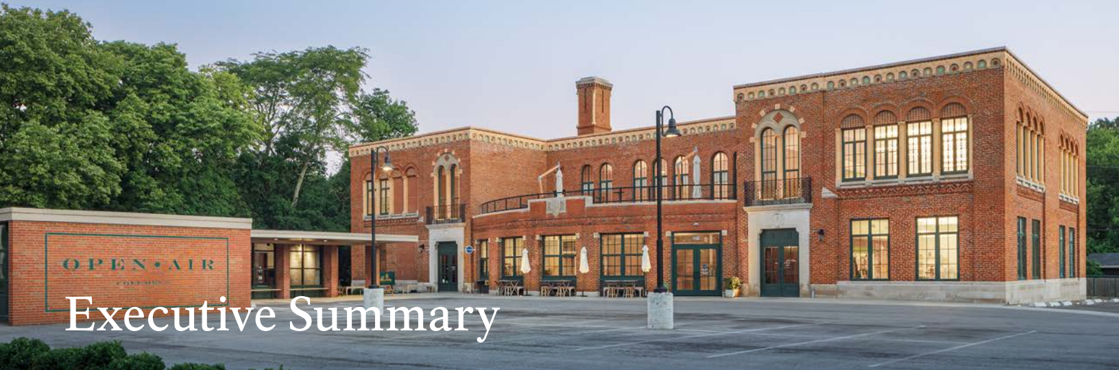
Open Air School, Columbus Ohio. Exterior after rehabilitation Photo: Kelley Companies
